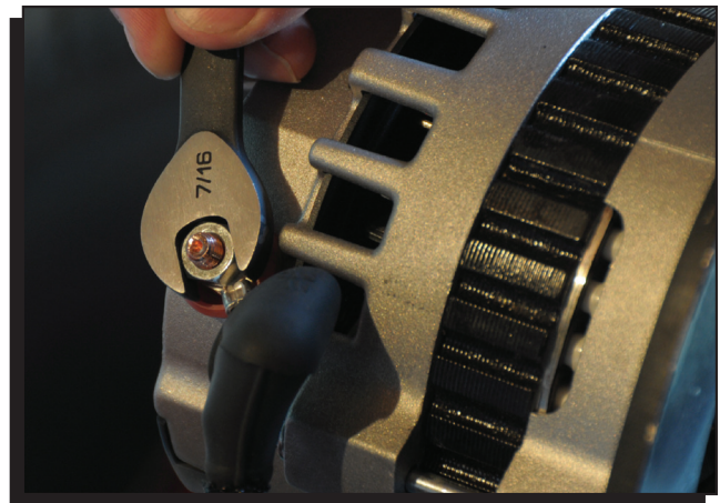
Figure 4 Installing the Charge Wire.
